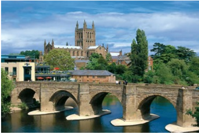
Hereford road bridge 33.9 miles
