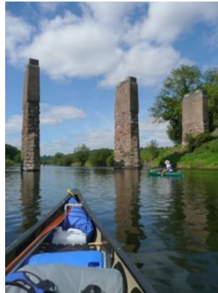
Demolished railway bridge CAREY 48.4 miles
