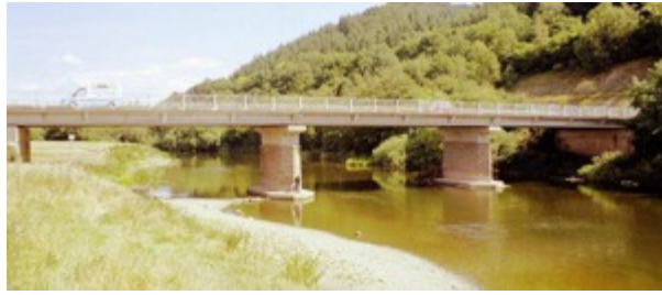
Even Pits/ Holme Lacy Bridge B4399 41.6 miles
