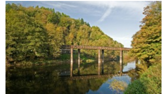
Redbrook old Rail Bridge 84.5 miles
